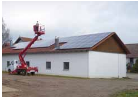
Specially trained staff performs measurements with a thermal imaging camera
